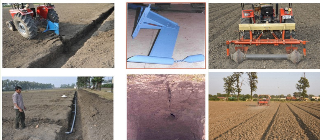
Fig. 1 Construction of Mole drains with sump well and BBFs
